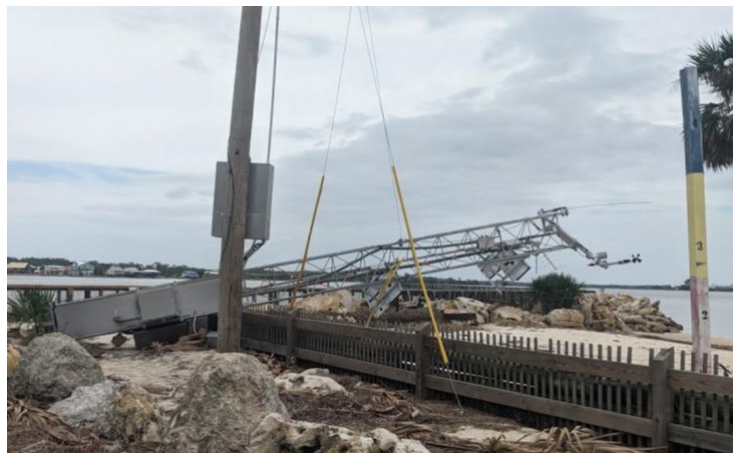
NOAA National Data Buoy Center station knocked down at Keaton Beach, Florida.
