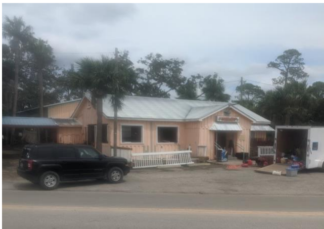
A Steinhatchee local said Idalia’s storm surge reached the top of this building, which sits directly across the street from the Steinhatchee River.
