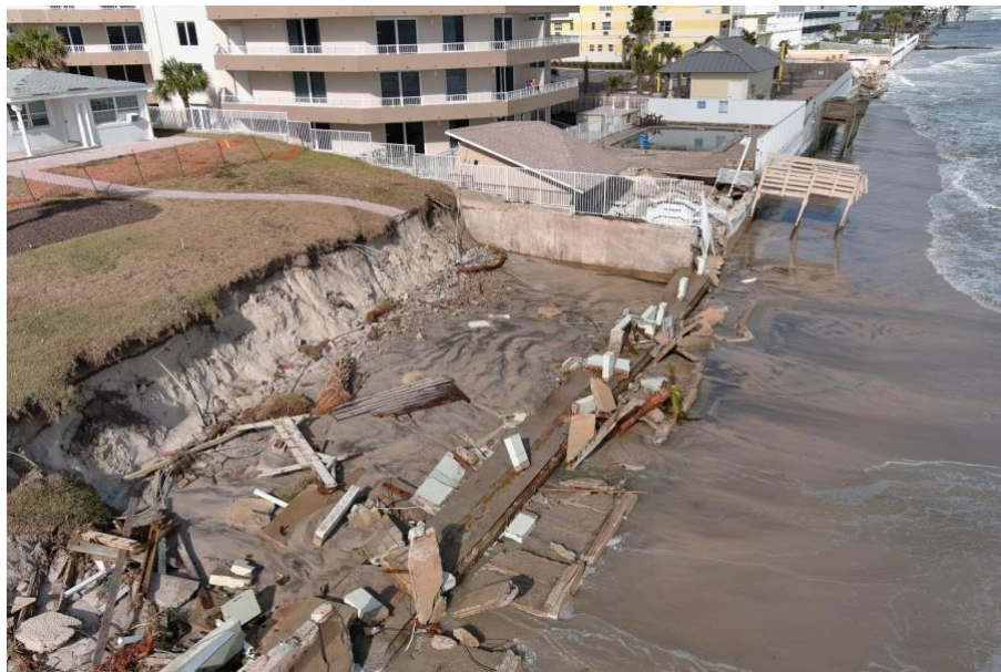
Figure 12. Beach damage and coastal erosion due to Hurricane Nicole in Volusia County (source: NWS Melbourne, credit: Volusia County).
