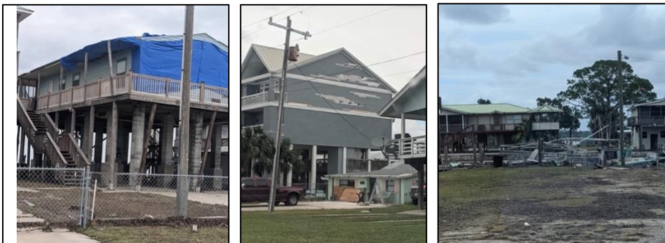
Damage to homes on Keaton Beach, FL, where Idalia made landfall on Aug. 30 as a category 3 storm.
